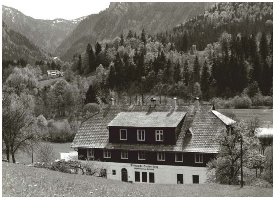
Fig. 93: Biological Station in Lunz
